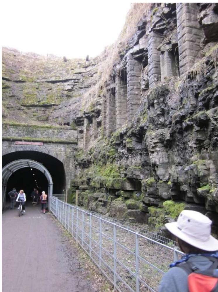
Figure 3 : Rampart supports to the Eyam Limestones in Headstone Tunnel cutting. Image: Patrick Cossey
